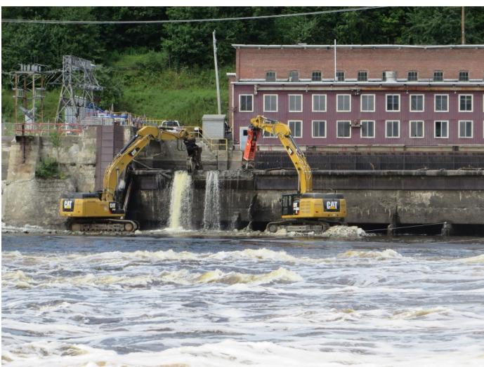
Removal of the Veazie Dam on the Penobscot River in Veazie and Eddington, Maine. More than 50 hydropower dams in the region are scheduled for relicensing in the next decade, requiring communities to make critical decisions about the future of dam infrastructure. Photo by Joshua Royte.
