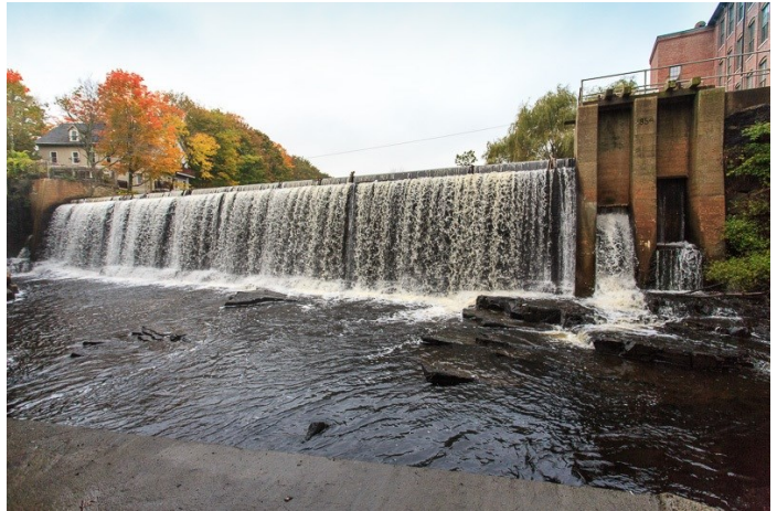
The Kesslen Dam on the Mousam River in Kennebunk, Maine. Iconic mill dams are an integral part of New England's industrial history and continue to provide some recreational, water supply, and aesthetic benefits for many communities. Photo by Ken Janes.
